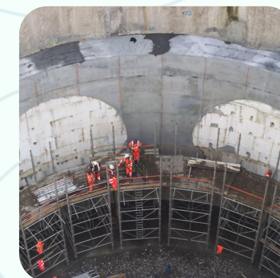
VOID FILL IN TUNNELS & CAVITIES
