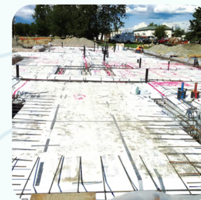
UNDER SLAB INSULATION
